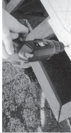
Carefully drill a 1/4" diameter hole just to the outside of the pattern at all corners where you're going to have to change direction while cutting. Make sure to wear safety goggles and don't do this without proper adult supervision.
